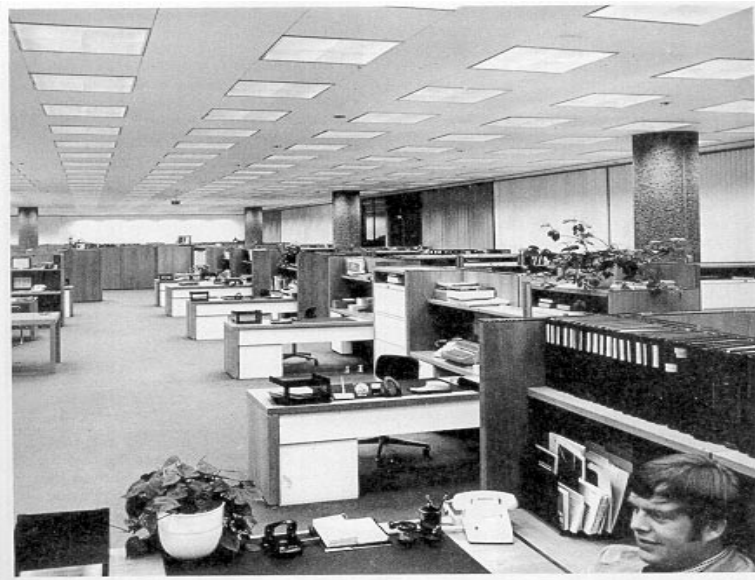
Figure 128—Two U-Shaped Fluorescent Lamps, with Efficient, Low-Brightness Anodized Aluminum Luminaire, Are Employed in Each Unit to Supply Lighting from the Ceiling
