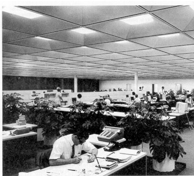
Figure 126—Ceiling System Providing Illumination, Air Supply, Air Return, Space Partitioning, and Acoustical Treatment
