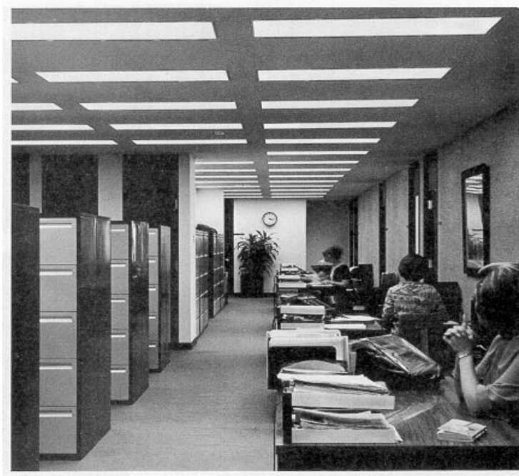
Figure 130—Secretarial Area with Uniform Lighting That Has Non-Uniform Possibilities
