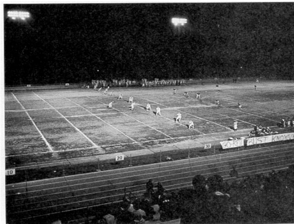
Figure 142—High School Football Field Lit with 1500 W Metal-Halide lamps
